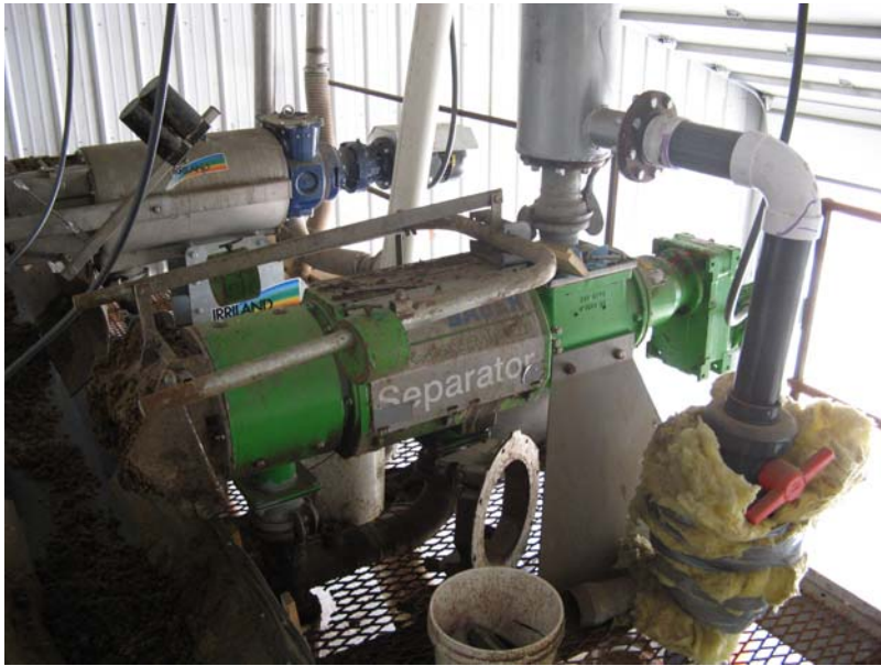
Screw-press separators
